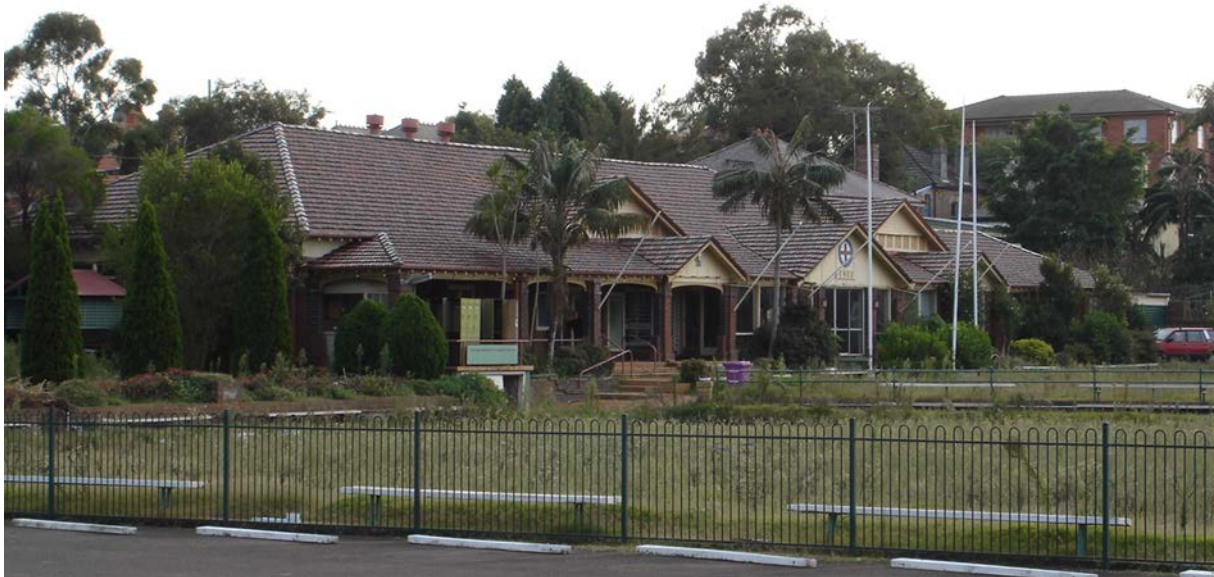
Figure 9: View of the former clubhouse from the Harrow Road car park
